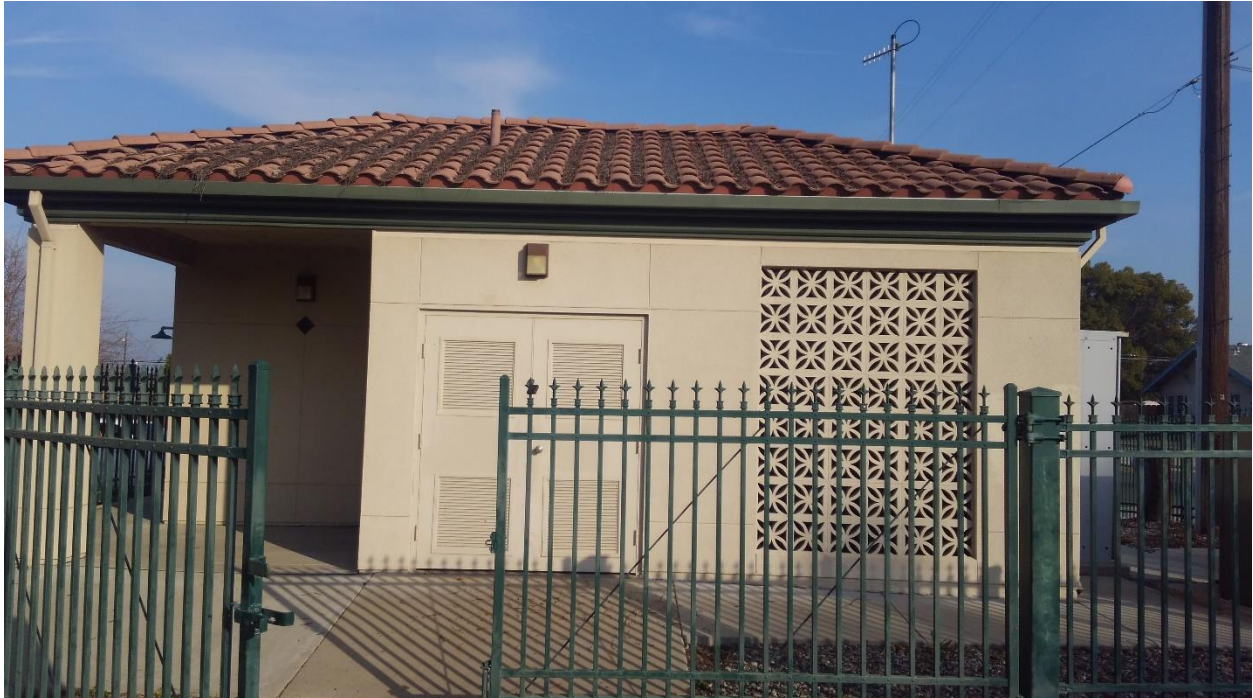
Figure 3a. Sample well site facility 1
